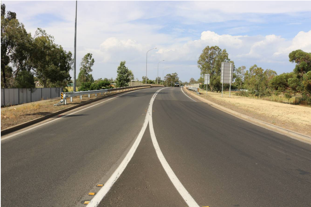
Photograph 3 – Kamilaroi Highway, near site.
